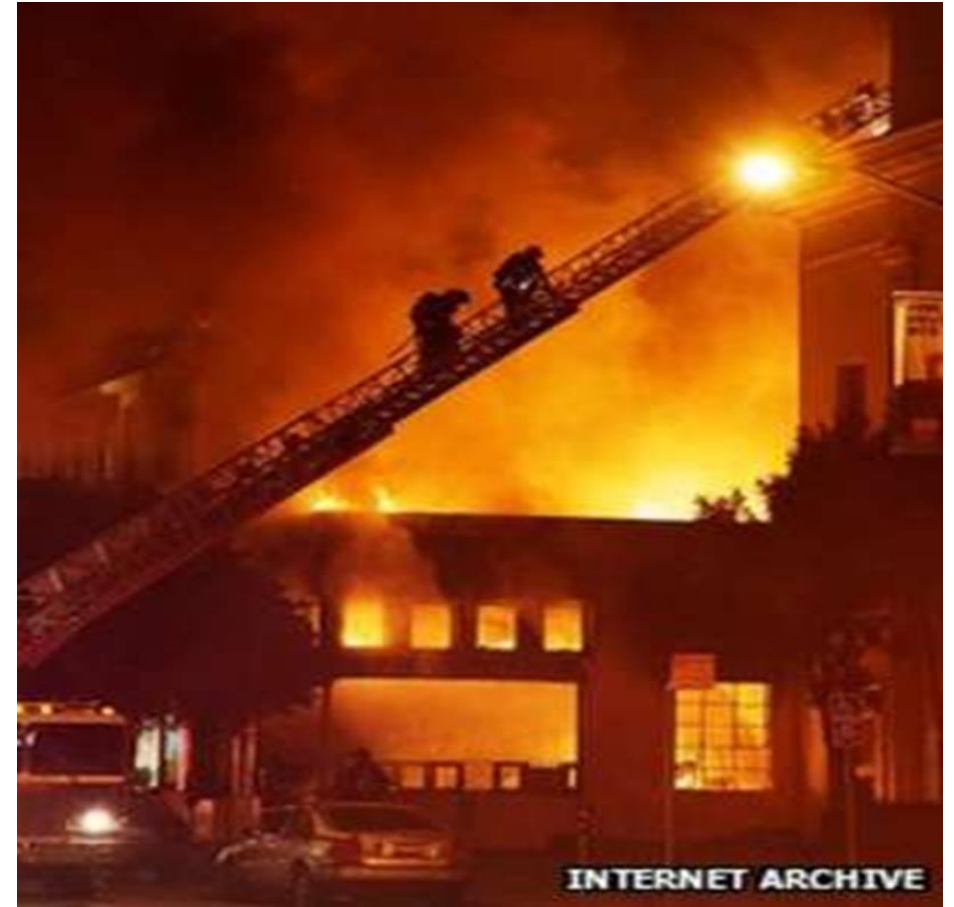
Internet archive building damaged by fire BBC news 7 November 2013
